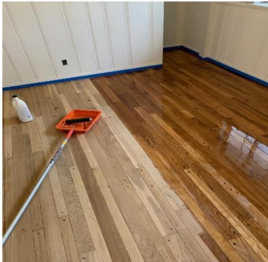
Fig. 1. Applying Tung oil to floor. Image obtained from Real Milk Paint
