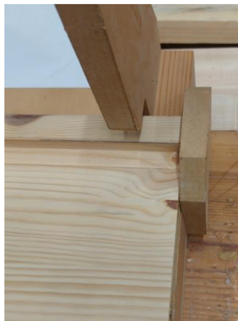
Note that ends are kept flush with MDF guide
