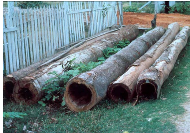
Figure 5: Termite damage in tropical hardwood poles
