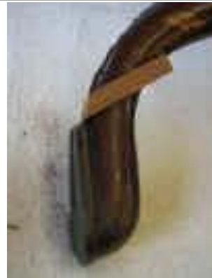
Missing section rebuilt
